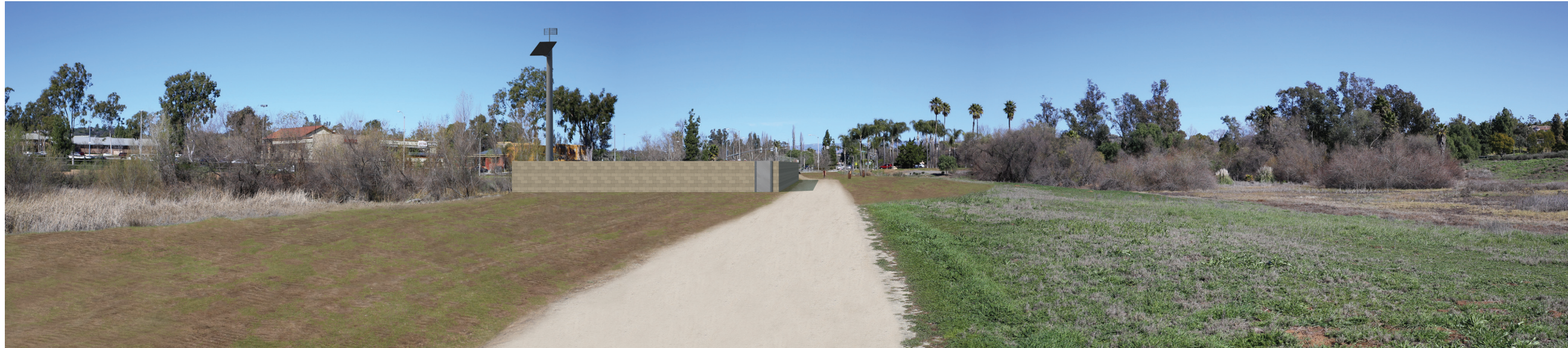
Visual simulation of the Proposed Project right-of-way as seen approximately one year after the completion of construction.
